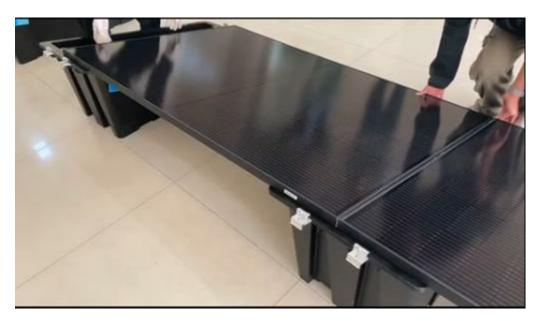
9. After confirming the position of the solar panel, tighten the screws on the clamps to fix it.
